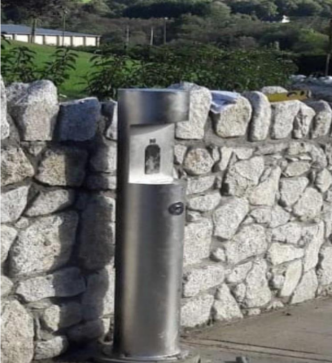
Water Refill Station installed at Rednagh Road, Aughrim
