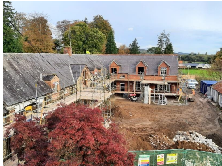
Construction of the Clermont Content Creation Enterprise Hub at Wicklow County Campus, Rathnew
