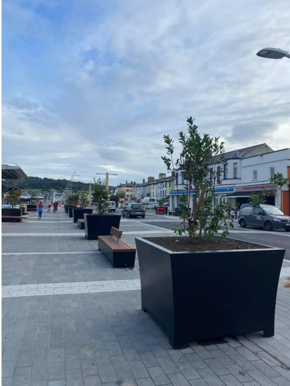
Seafront Plaza works completed
