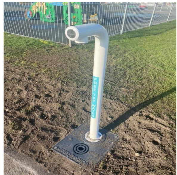
Drinking water fountains installed
