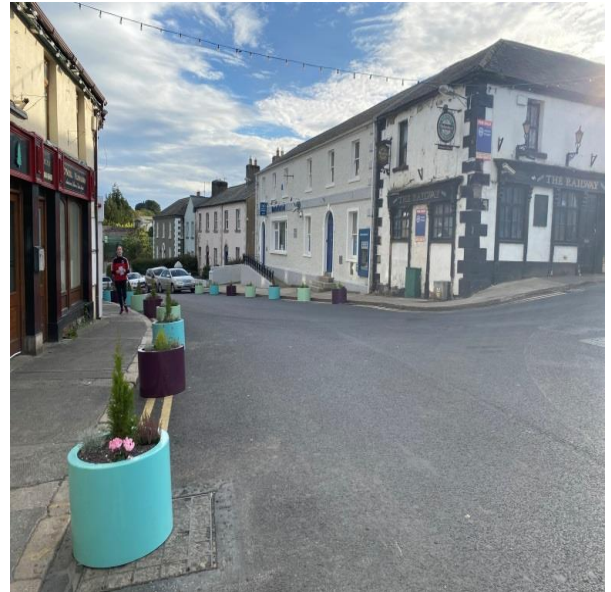
Rathdrum Main Street Enhancement Scheme
